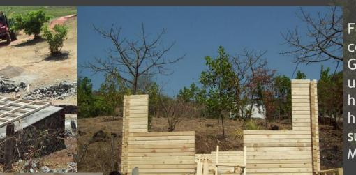
For a very Brief Period we developed and started construction of Single Panel T&G (Tongue & Groove) houses it was very short lived as we understood that these were not suitable for hotter climate conditions due to lack of insulation however here are some projects which weren't as successful due to the hotter climatic conditions of Maharashtra.
